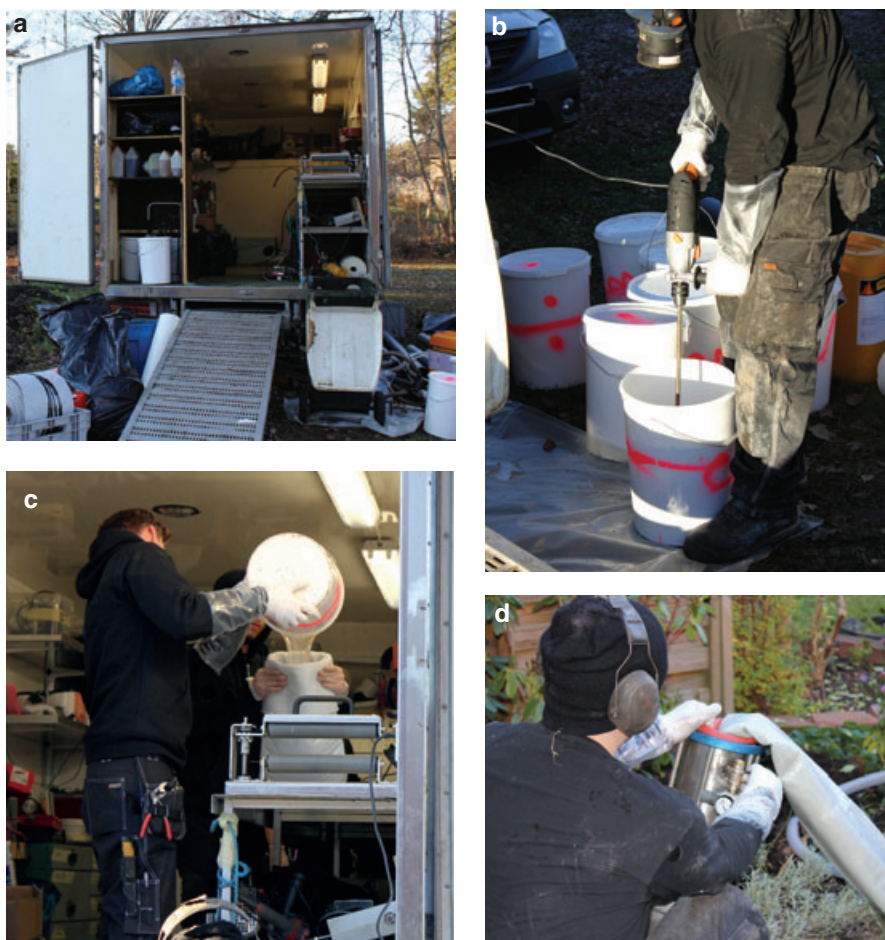
Fig. 1. The photographs show epoxy pipe relining work: a temporary worksite (a), a worker mixing the epoxy resin systems (ERSs) with the bucket between his feet (b), one worker holding the liner and the other worker pouring the mixed ERSs into the liner (c), and a prepared liner being inserted into the inversion drum (d).
