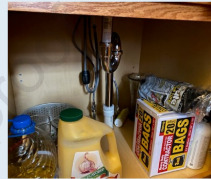
Leaky Plumbing Replaced - After
