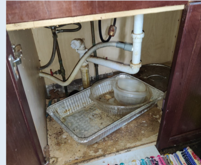
Leaky Plumbing Replaced - Before
