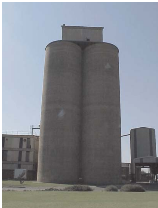
Maize silos at one of the mills.
