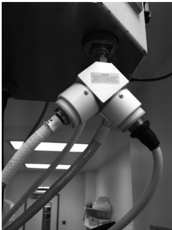
Figure 3 A suction splitter and suction outlet socket.
