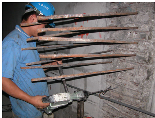
Fig. 2. The workers wore T-shirt and trousers without good protection from the epoxy resin systems during work.
